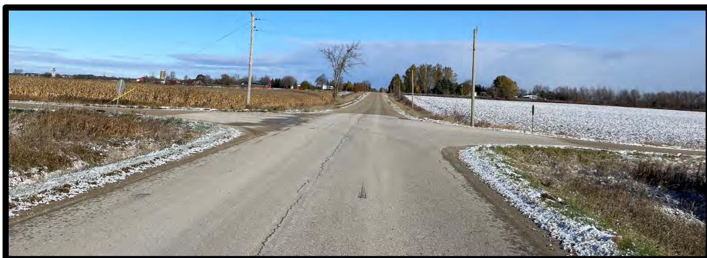
Picture 7 – Concession Road 4 North at Sideroad 6 E (November 1, 2023)
